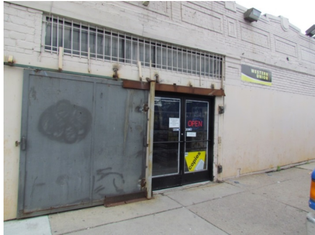
Photo # 26 – Storefront with Signage
